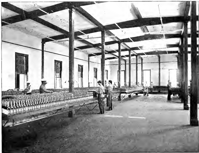
A room in the Bottling House, where Poland Water is Labeled.
